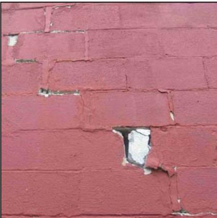
*This is an exterior view of a gaping crack in the masonry of Storage Bay #2. Pamela Ames photo*
