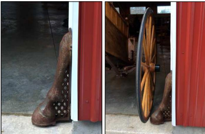
*This is a fancy Cast Iron Door Guard in the form of a horse's leg. It prevents the wheel from passing too close to the stable door frame thus avoiding the hub from fetching up.*
